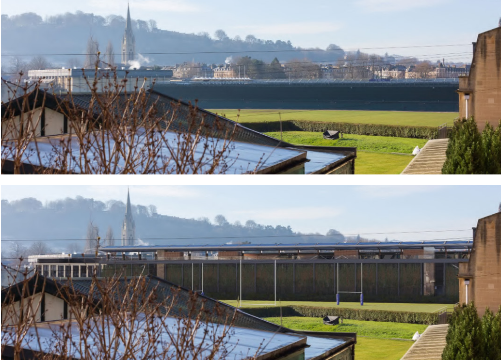
FIGURE 6 Verified “before and after” views of the proposed East Stand proposal as seen from the Rec. Note that the existing stand in the top image is temporary and is regularly disassembled for portions of the year.
